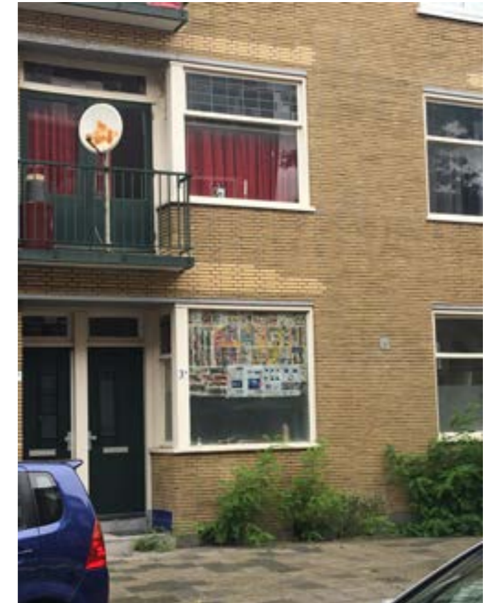
Figure 2: Bad treatment of the housing by inhabitants, 03-09-2019, Tarwewijk, Rotterdam, The Netherlands
